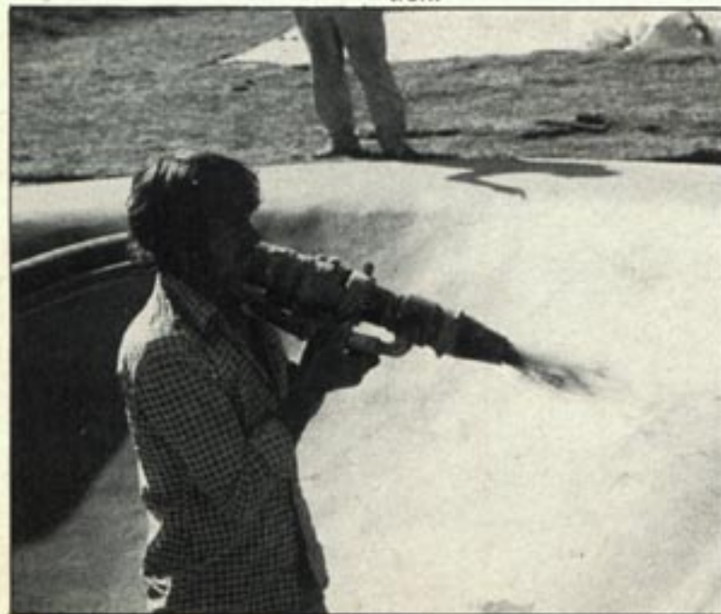
Top: Essential for any park, properly schemed landscaping. Above: Float-work on the newly-applied shotcrete. . . the half pipe takes shape. Below Left: A shotcrete application to the half pipe. Below right: The designers and builders, Adrian Rolt and Tony Wynne of G-Force and Skatepark Construction.
