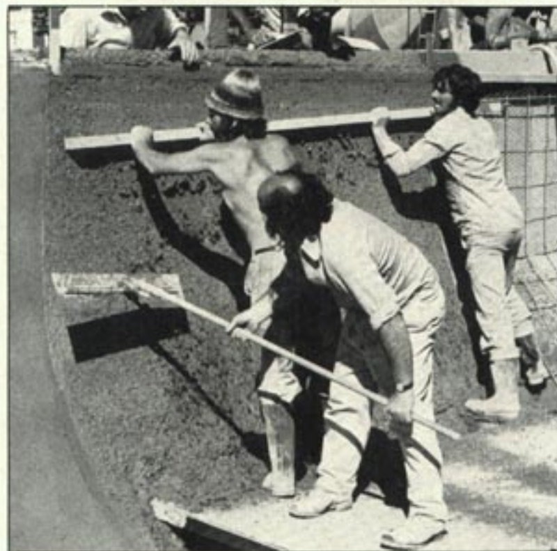
Top: Essential for any park, properly schemed landscaping. Above: Float-work on the newly-applied shotcrete. . . the half pipe takes shape. Below Left: A shotcrete application to the half pipe. Below right: The designers and builders, Adrian Rolt and Tony Wynne of G-Force and Skatepark Construction.
